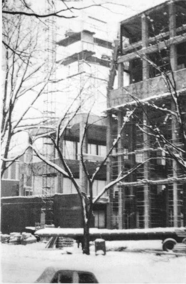
The Fine Arts building under construction.
